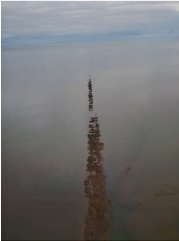
Figs. 1 and 2. Aerial photographs of the rock armoured Rossall outfall that extends for 5.2 km illustrating the height of the obstruction and the effects on tidal flow. Photographs taken above shore at Rossall looking west. 31 st August 2011.
