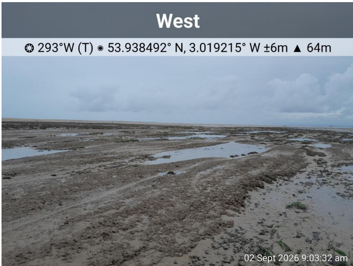
Figure 6. Persisting mussel mud and evidence of scour on Perch Scar
