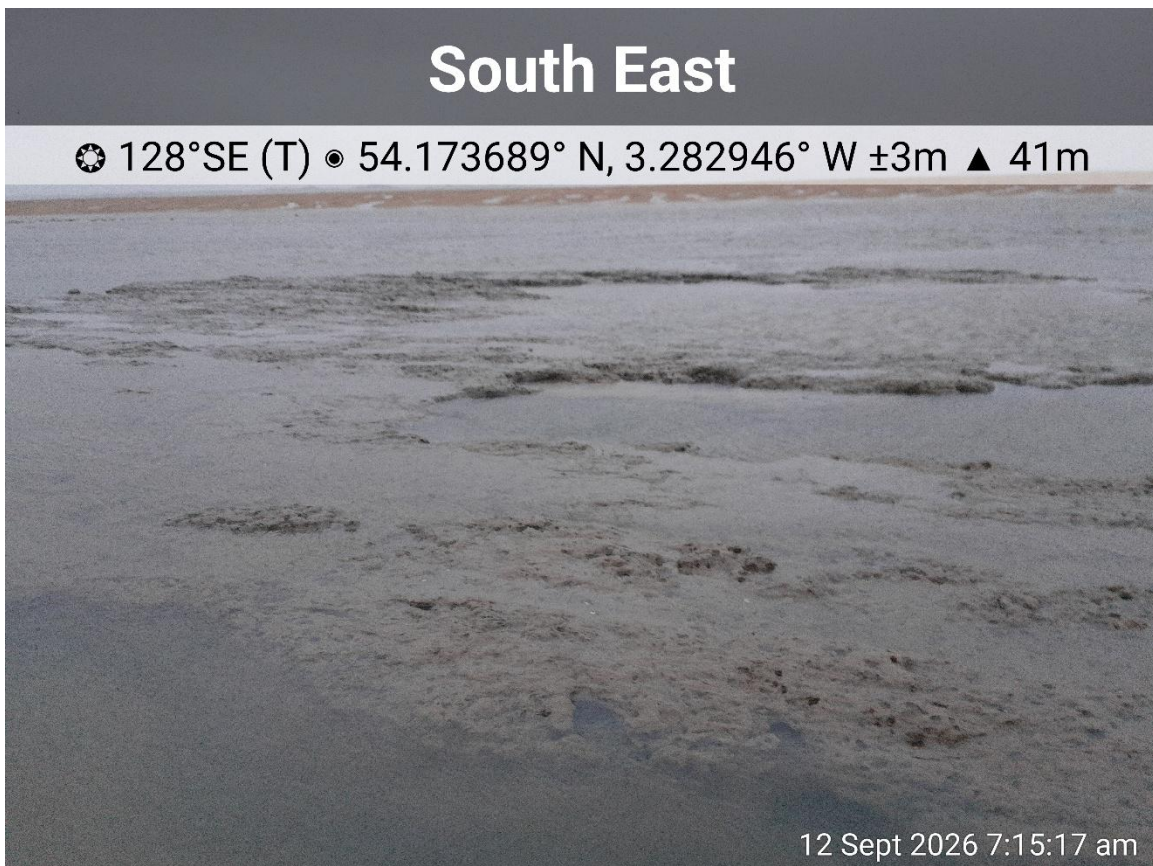
Figure 4 (b) Large patches of scour approximately 2ft deep
